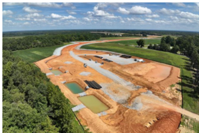
ASM mine site preparation
