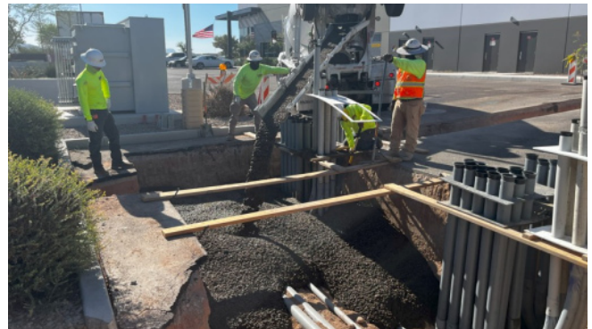
Urbix pilot production facility construction
