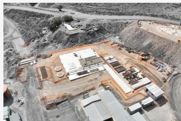
New water treatment plant under construction
