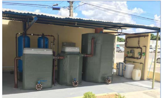
New Water Treatment Plant in União Baiana
