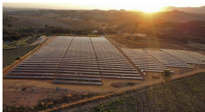
One of Omnigen's solar power plants
