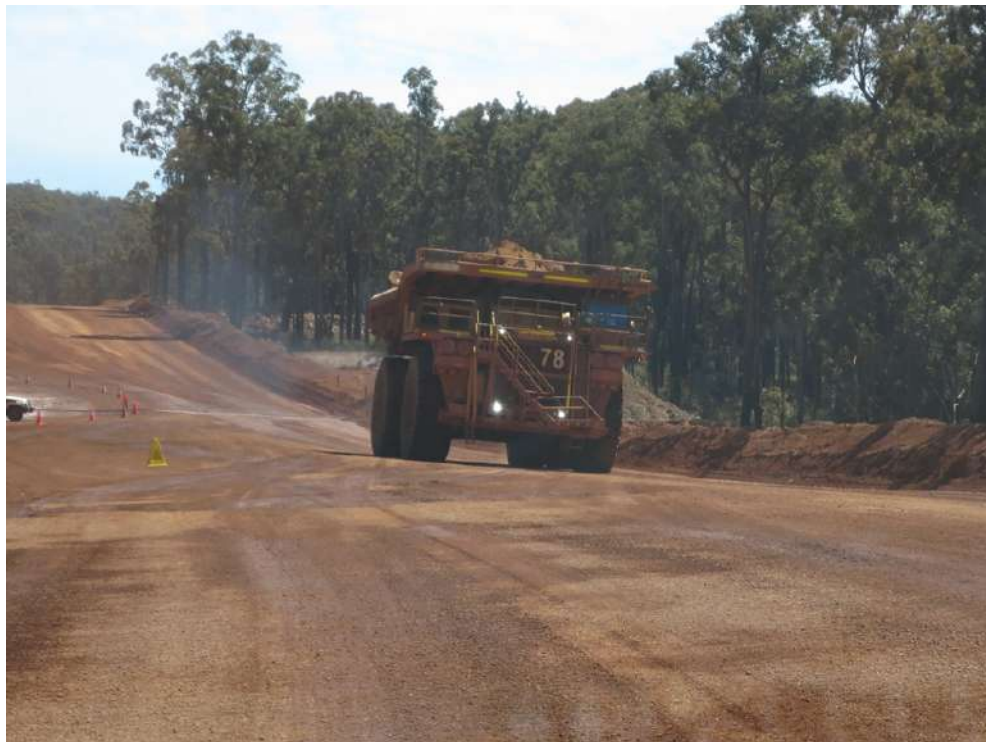
Figure 13-5: Haul Roads with Berms (SLR, 2021)
