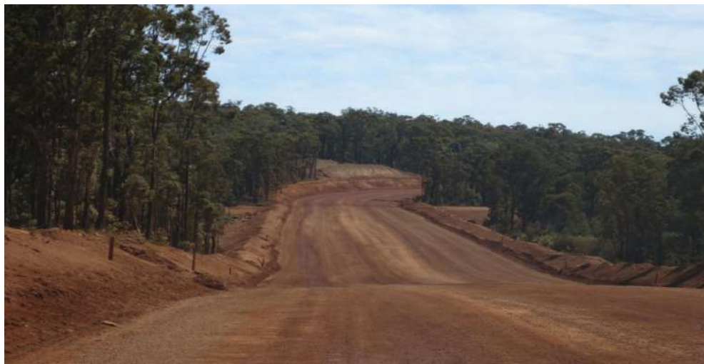
Figure 13-5: Haul Roads with Berms (SLR, 2021)
