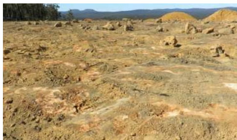
Top soil and oxalate removed leaving Hardcap
