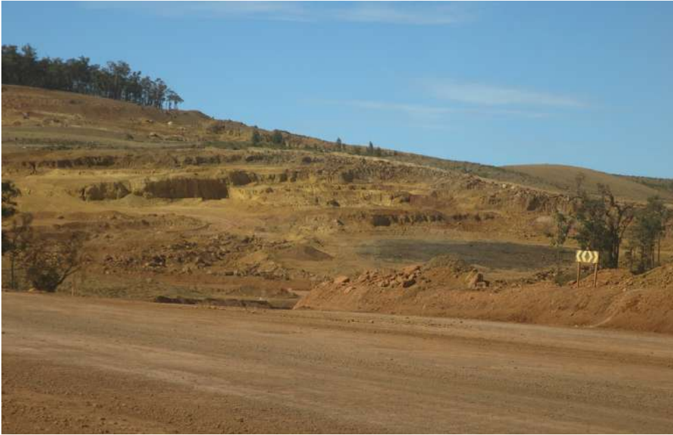
Figure 13-8: Soil Being Returned for Backfilling and Landscaping the Pit (Alcoa, 2018)
